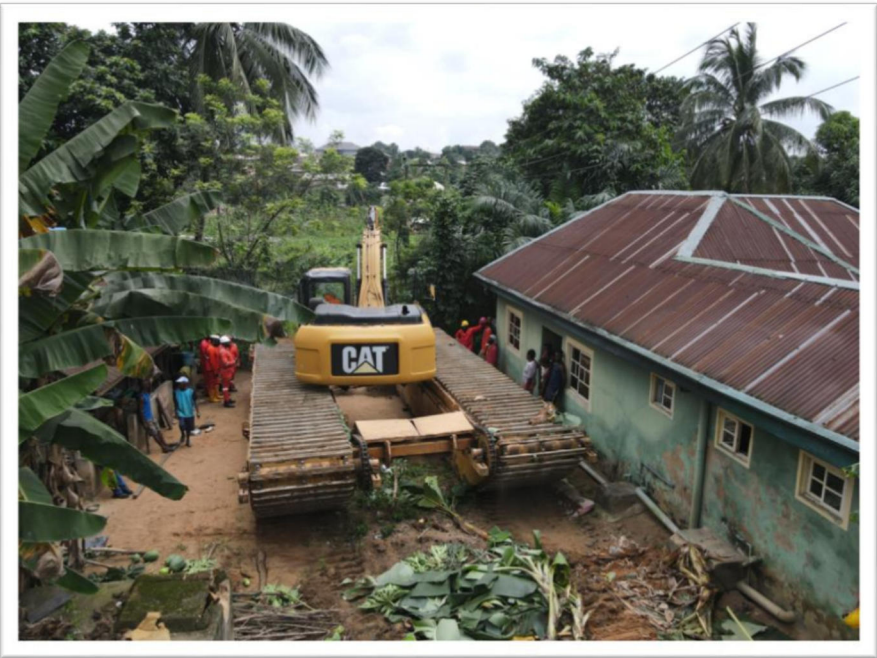
Nigeria Breweries Trenching
