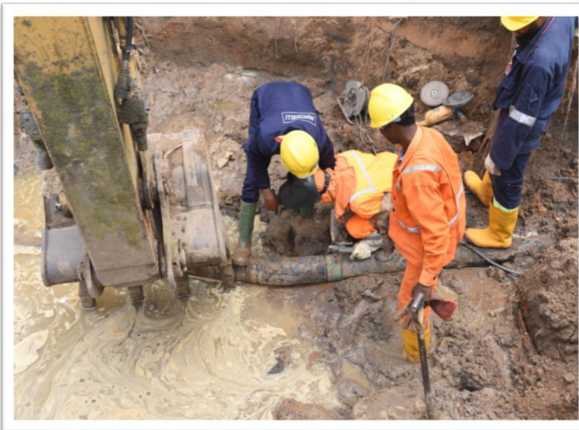
Nigeria Breweries River Crossing Tie-in 1
