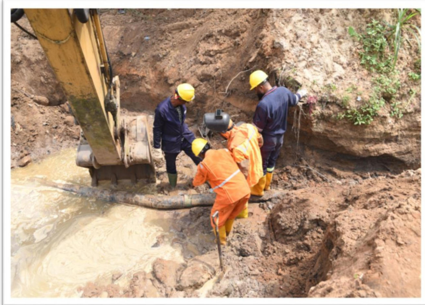
Nigeria Breweries River Crossing Tie-in
