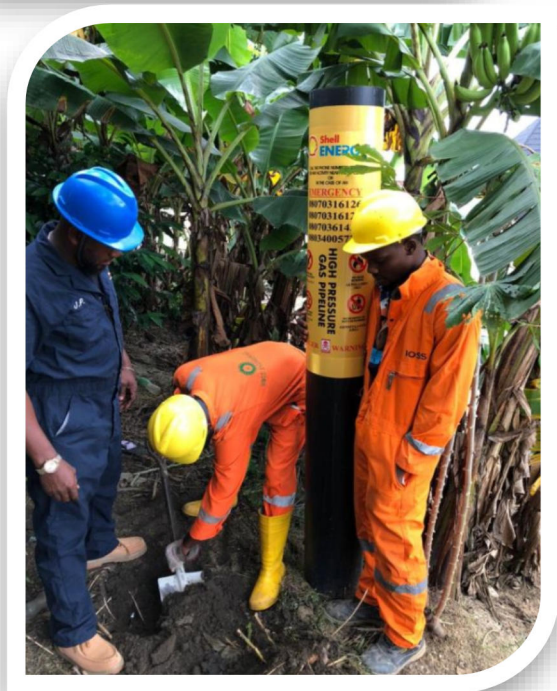
Selected Pictures of On-going Projects UPVC route marker installation
