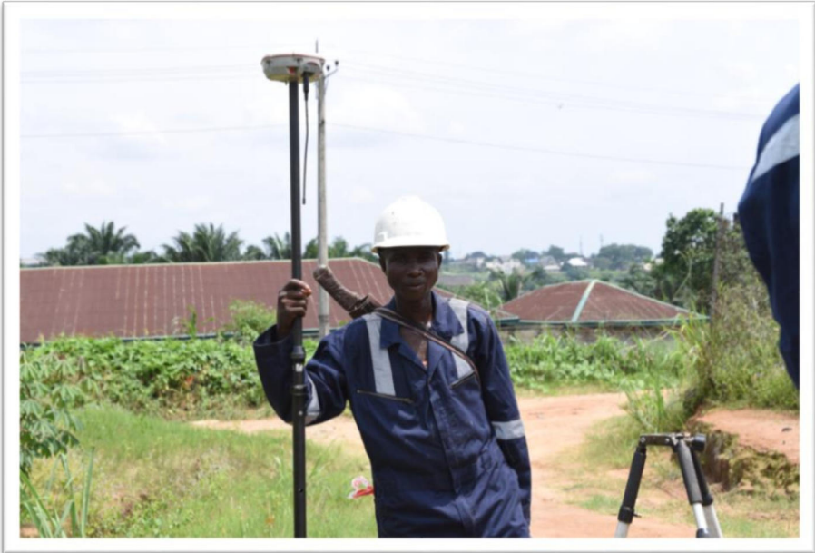
Nigeria Breweries Survey in Progress
