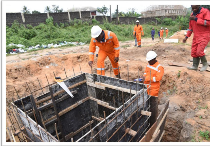
Nigeria Breweries Line Break Valve Pit Formwork
