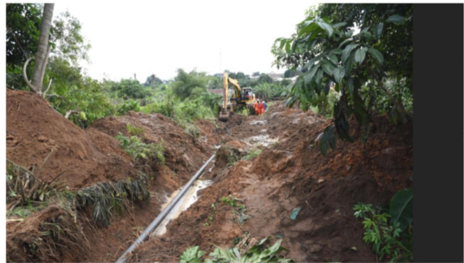
Nigeria Breweries Pipe Stringing 1
